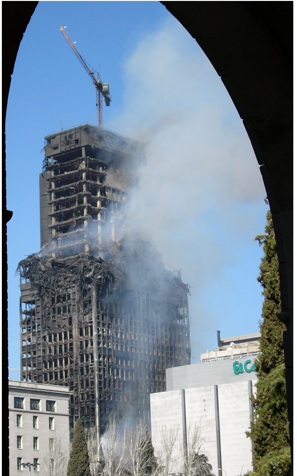
Photographer: Manuel González Olaechea y Franco. The building is still strong enough to support the crane on top.
