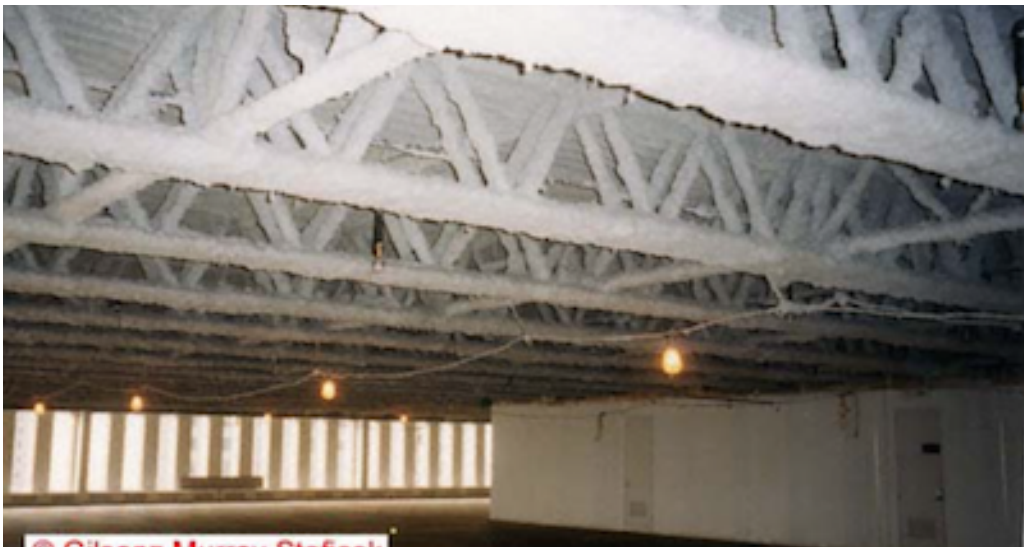
A photograph of WTC trusses with fireproofing
