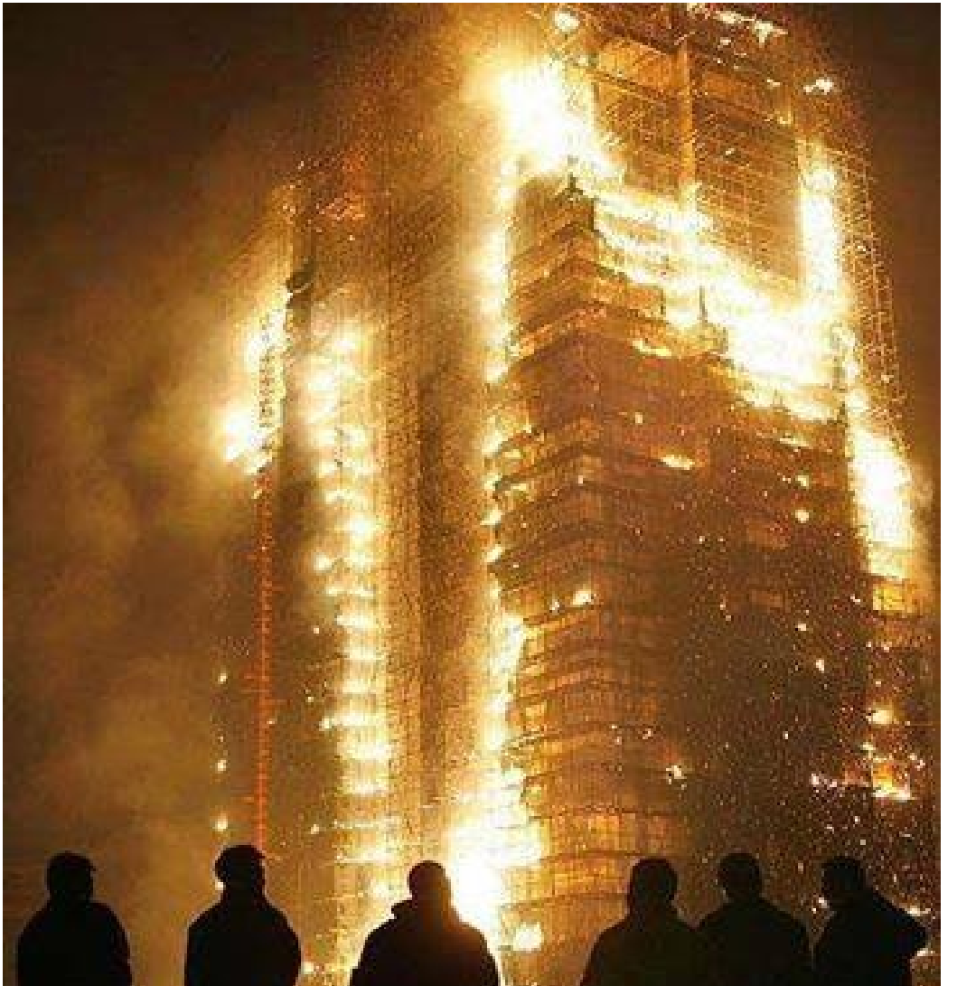
The Windsor tower in Madrid burned for 24 hours and had no fireproofing on the steel.
