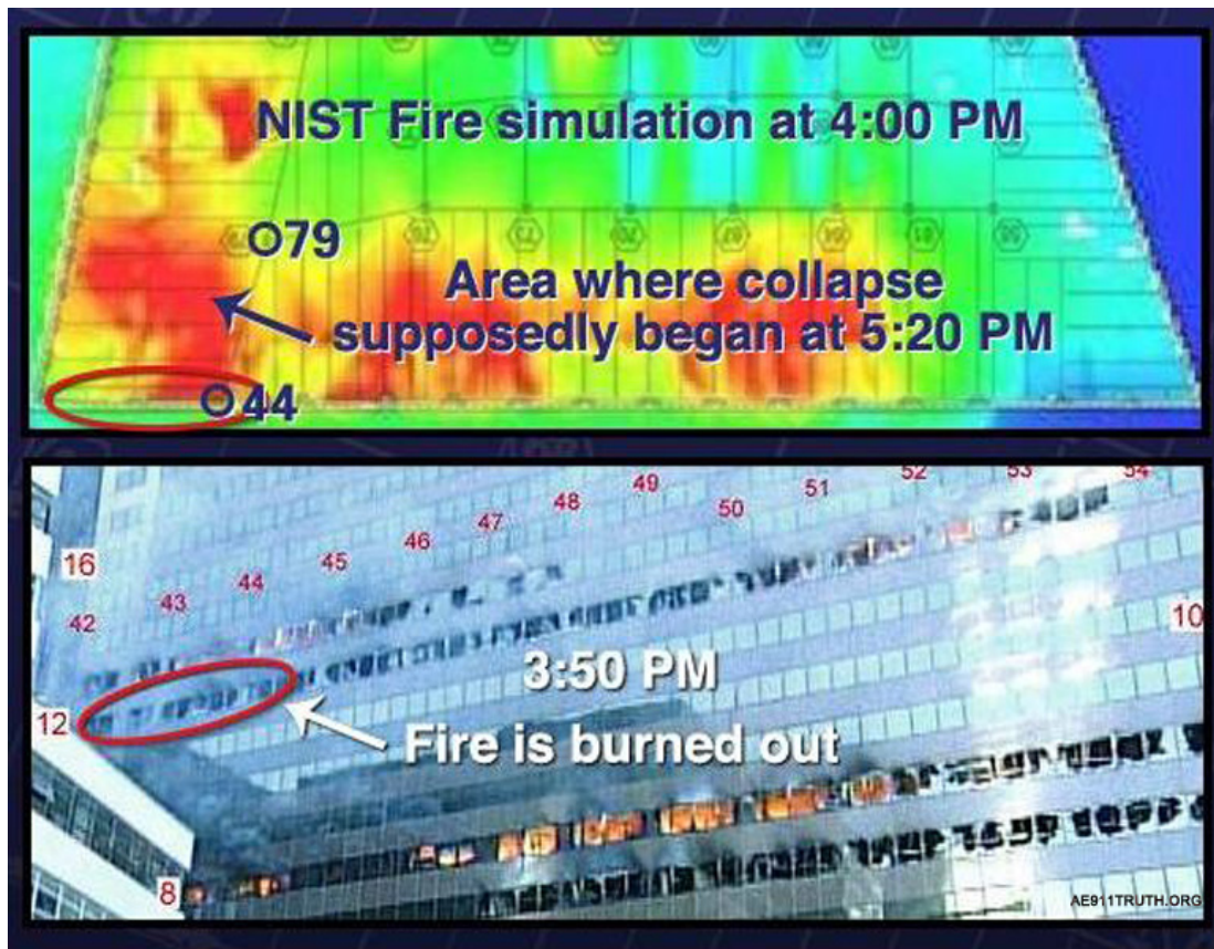
Figure 11. According to NIST, a fire on the northeast corner of WTC 7's Floor 12 (see red oval in both frames above) thermally expanded the floor beams of the floor above it, triggering the collapse of Building 7 at around 5:20 PM on 9/11/01. In the top frame, NIST's computer-based fire "simulation" shows a raging fire in this location at 4:00 PM. But in the bottom frame, NIST's photographic evidence shows that the fire in the critical area had burned out before 4:00 PM (see NCSTAR 1-9 Vol. 1, Figure 5-136).
